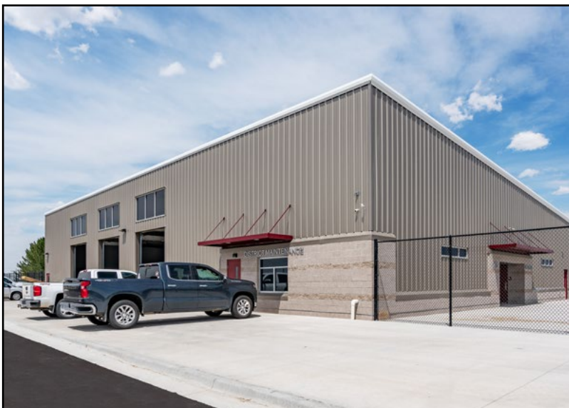
Brush School District Transportation Facility-
